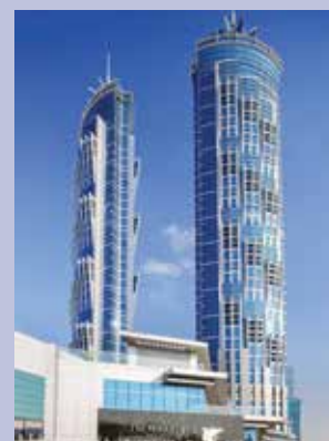
PIC: JW MARRIOTT MARQUIS HOTEL DUBAI
