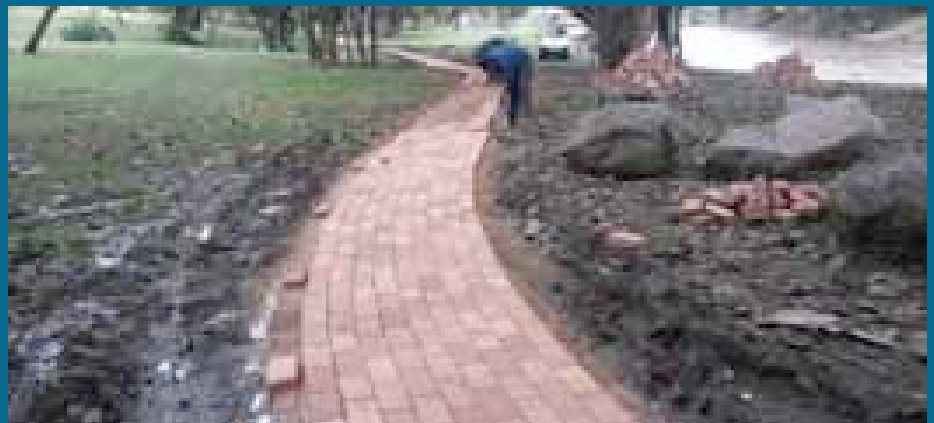
Paving in progress
