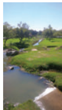
Cutting of reeds in waterway at Phase 2 has been completed
