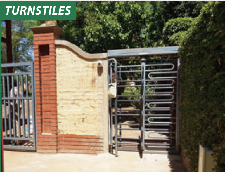
The turnstile was moved and a new entrance was done for the Contractors and Domestics.
