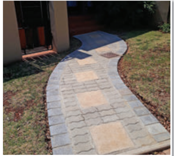
New Pathways are being laid leading to the front doors.
