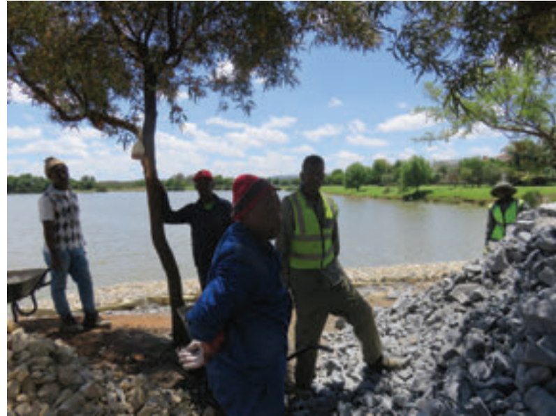
Staff building the gabions
