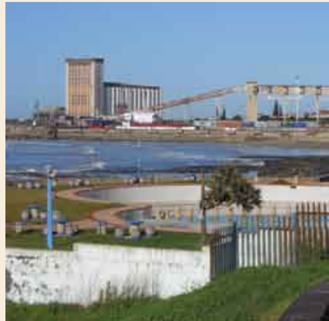
East London is to benefit from a R20-million refurbishment of the port's grain elevator.
