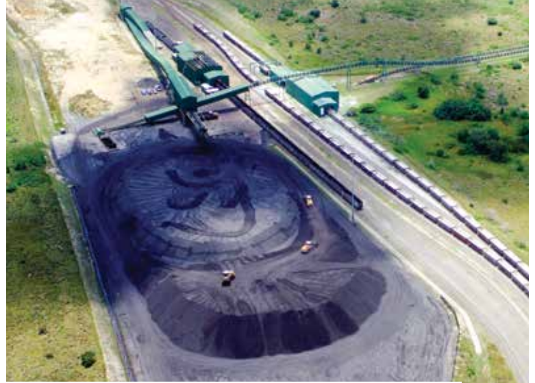
An aerial view of the Richards Bay coal terminal. Photo: Grindrod
