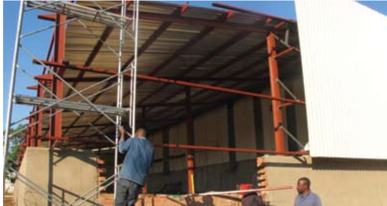
SDV's newly upgraded warehouse ... already operating at near-capacity.
