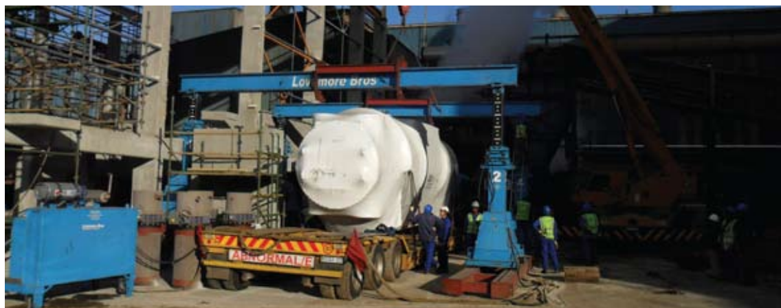
The Lovemore Bros lowbed arrives at the Royal Swaziland Sugar Corporation's mill at Simunye to install the generator and condenser which its lowbeds transported from Durban harbour.
