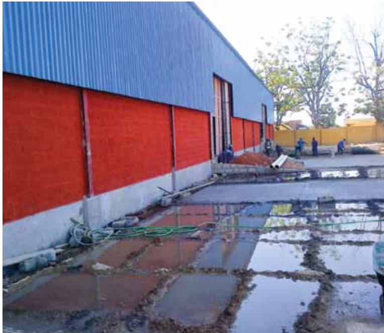
Bollore's new warehouse under construction in Lusaka.
